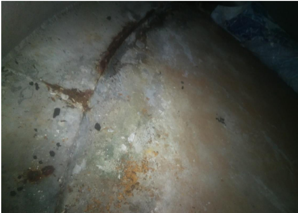
Photo 18: Annular plate was observed with minor rusting.
