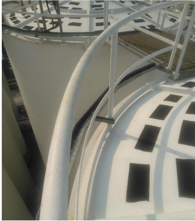
Photo 29: Roof handrail and joints were in satisfactory condition
