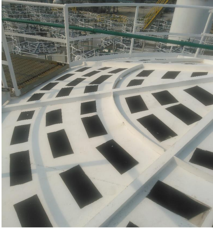
Photo 27: Roof plate was observed in satisfactory condition.
