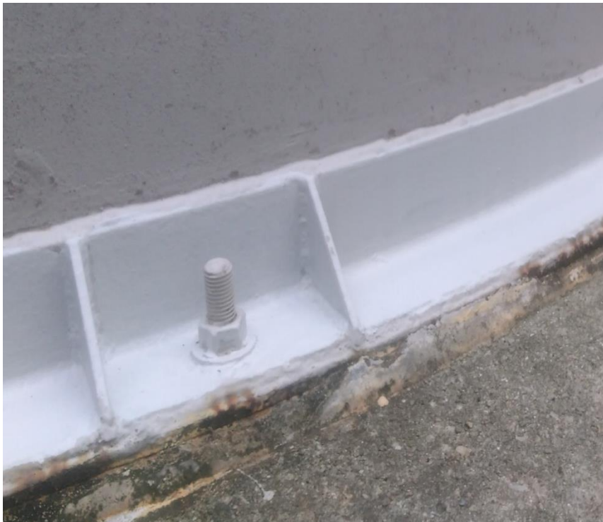
Photo 6: Bottom angle ring, bolts & grouting were in satisfactory condition.
