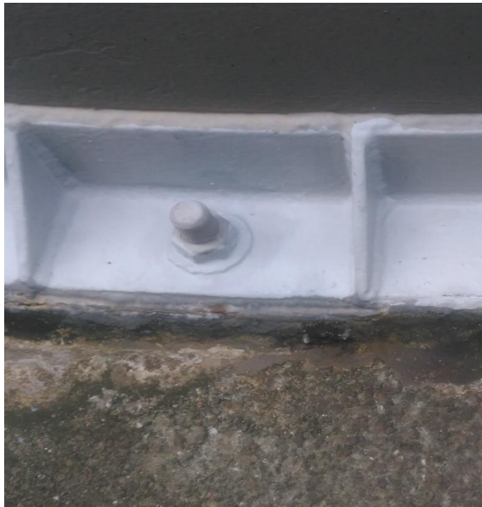
Photo 10: Bottom angle ring, bolts were in satisfactory condition. Damaged grouting was noted.
