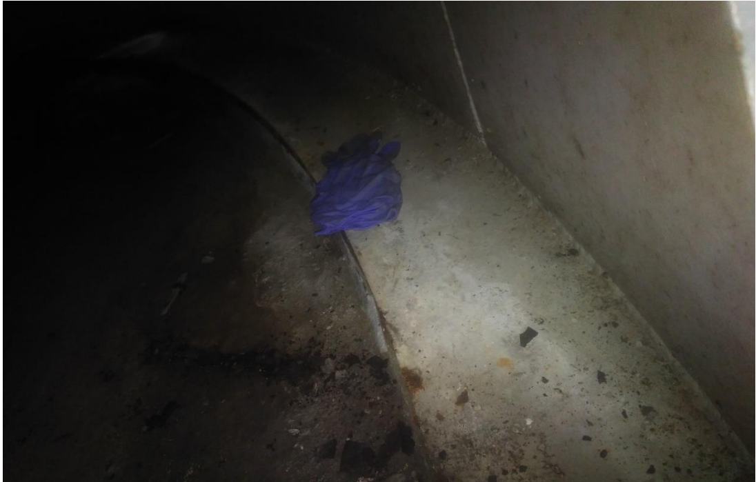
Photo 19: Annular plate was observed with minor rusting.
