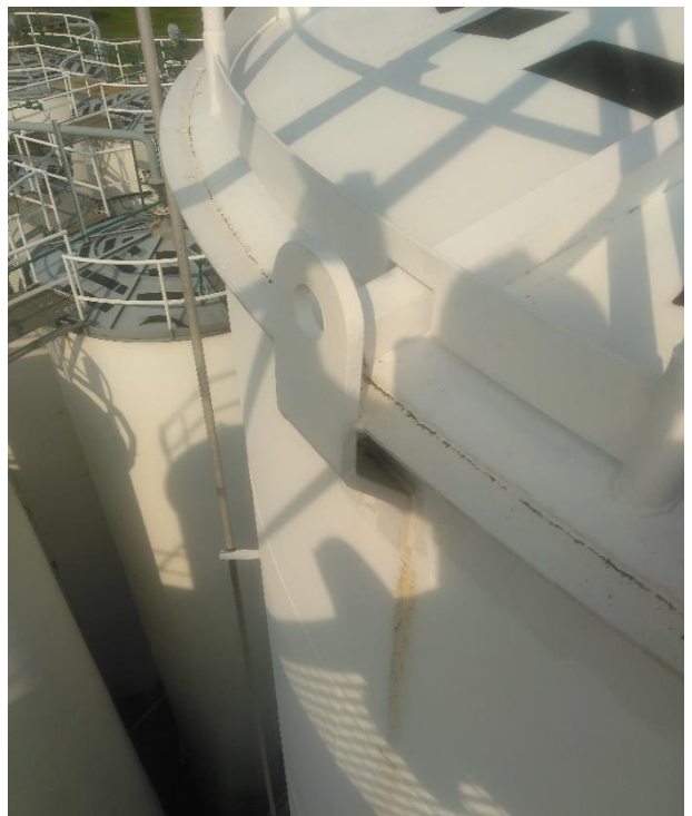
Photo 36&37: Top angle ring and lifting lug were in satisfactory condition
