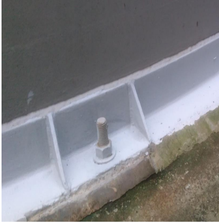
Photo 9: Bottom angle ring, bolts were in satisfactory condition. Damaged grouting was noted.
