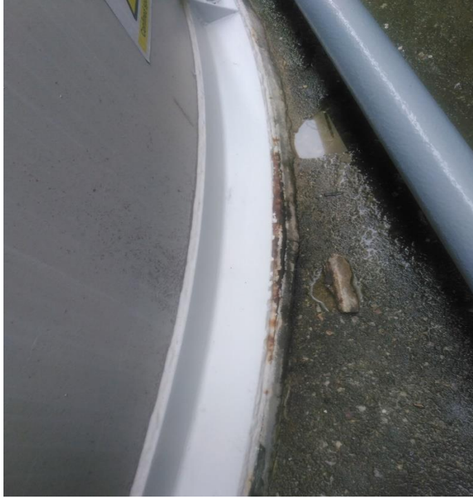
Photo 11: Bottom angle ring, bolts were in satisfactory condition. Damaged grouting was noted.
