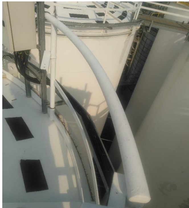
Photo 30: Roof handrail and joints were in satisfactory condition
