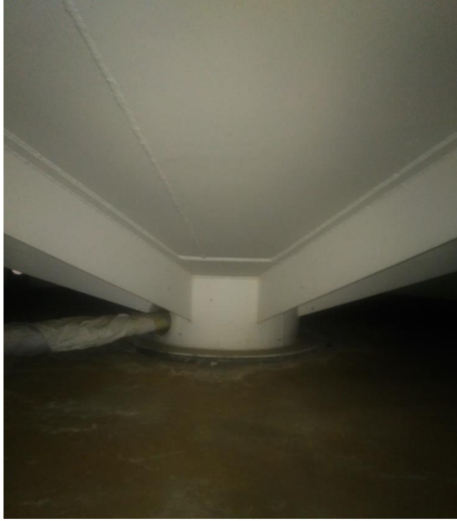
Photo 17: Bottom cone was observed satisfactory condition.
