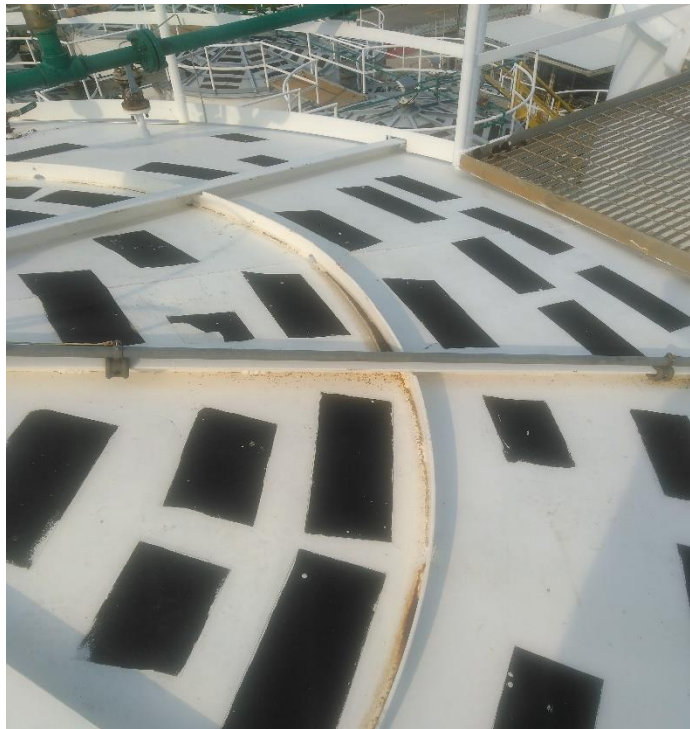
Photo 28: Roof plate was observed in satisfactory condition.
