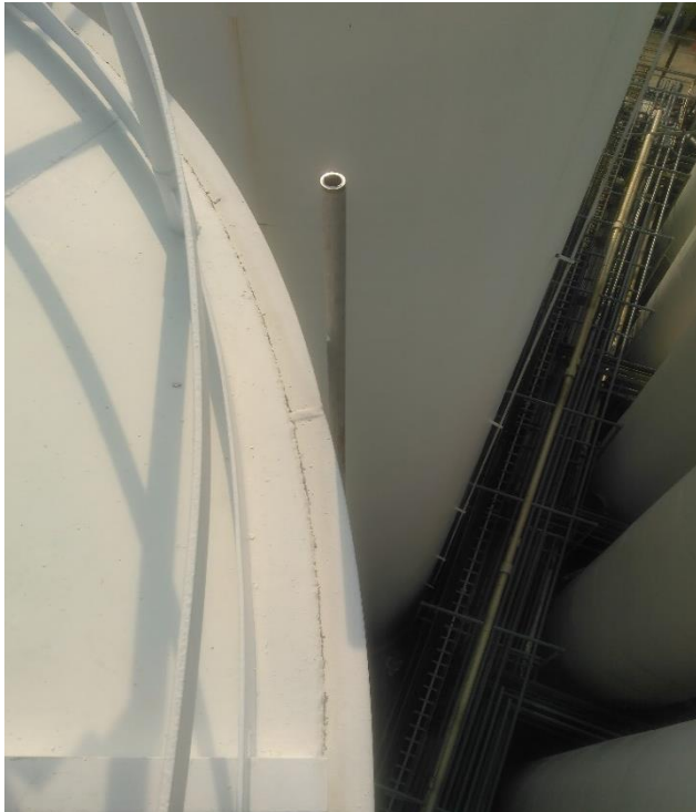
Photo 36&37: Top angle ring and lifting lug were in satisfactory condition
