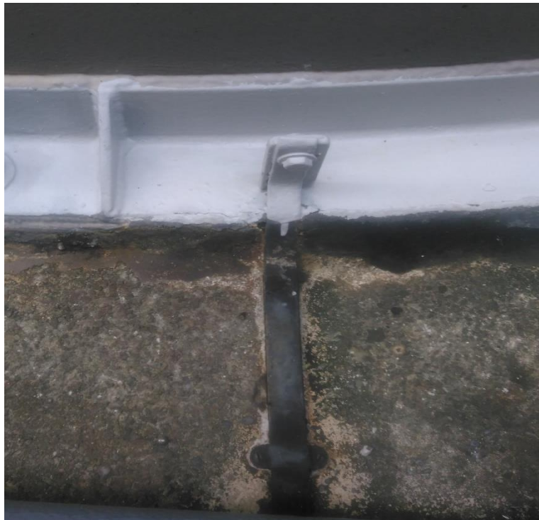
Photo 20: Earth cable was observed satisfactory condition.
