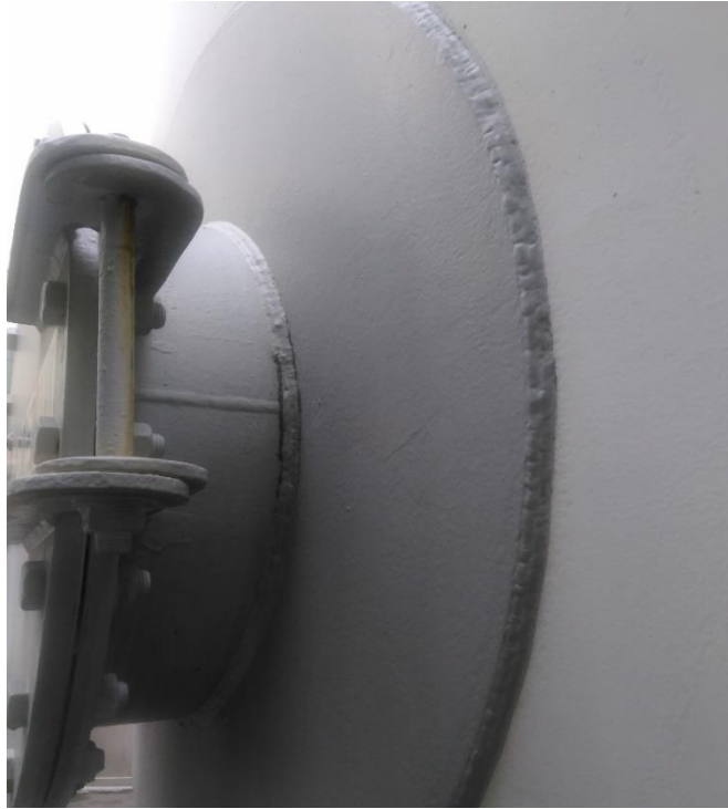
Photo 13: Manhole, reinforcement plate were observed in satisfactory condition.
