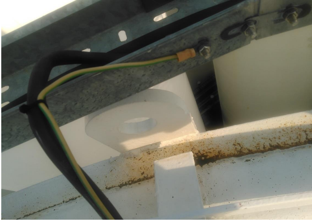
Photo 35: Top angle ring and lifting lug were in satisfactory condition
