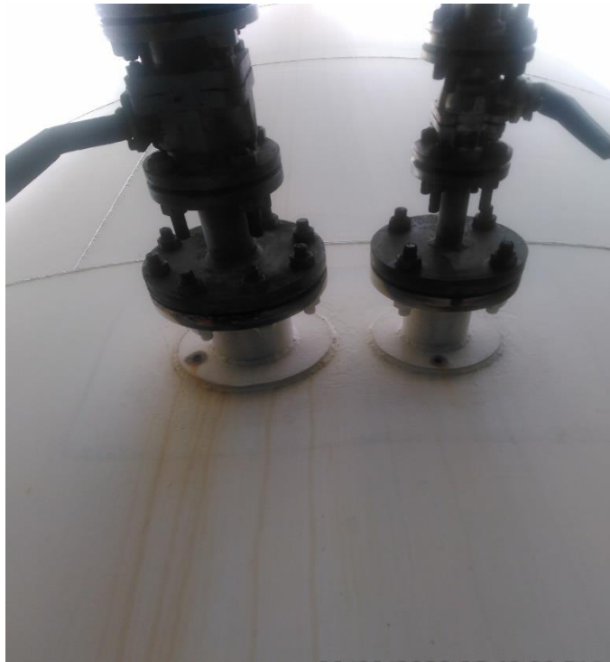
Photo 24: Remaining shell courses & nozzle was observed satisfactory condition
