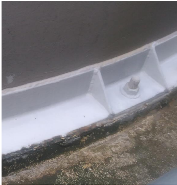
Photo 7: Bottom angle ring, bolts & grouting were in satisfactory condition.
