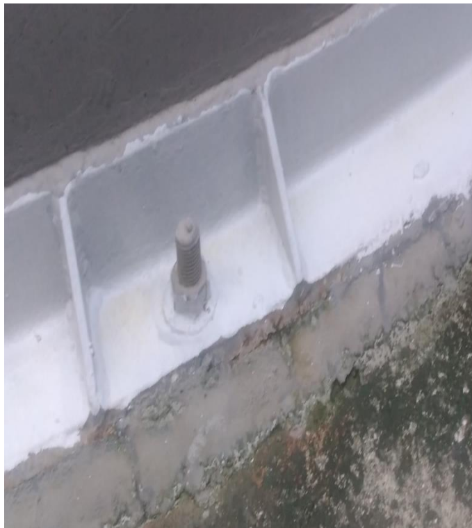
Photo 8: Bottom angle ring, bolts & grouting were in satisfactory condition.
