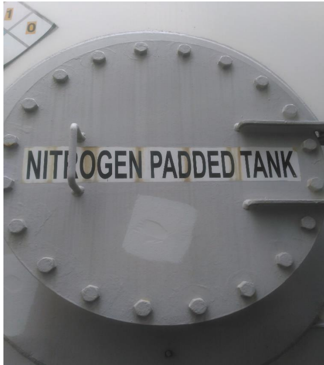
Photo 14: Manhole, reinforcement plate were observed in satisfactory condition.
