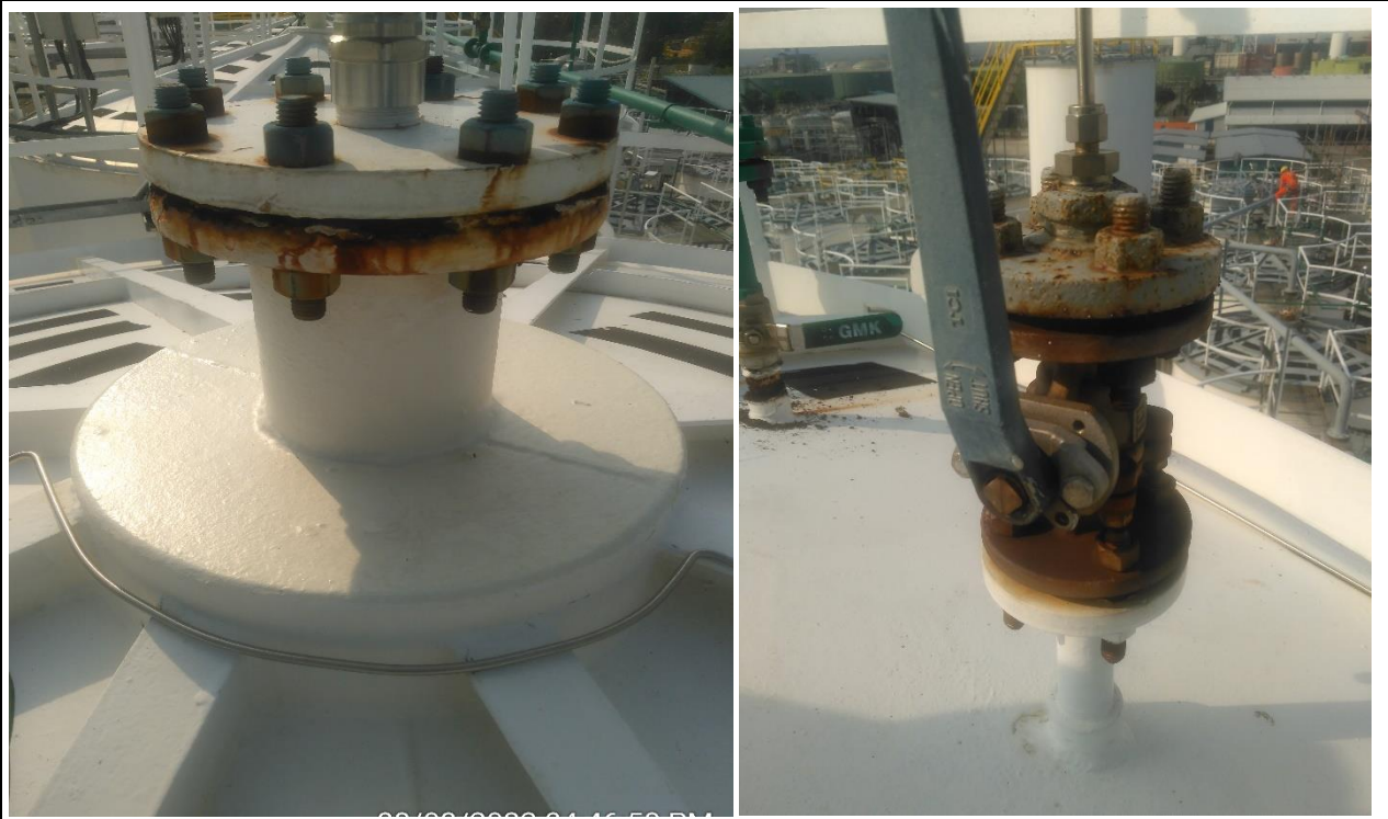
Photo 31&32: Roof nozzles and joints were in satisfactory condition.
