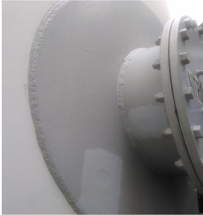
Photo 15: Manhole, reinforcement plate were observed in satisfactory condition.
