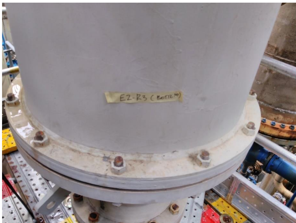
Photo 6: Shell & bottom channel were in satisfactory condition
