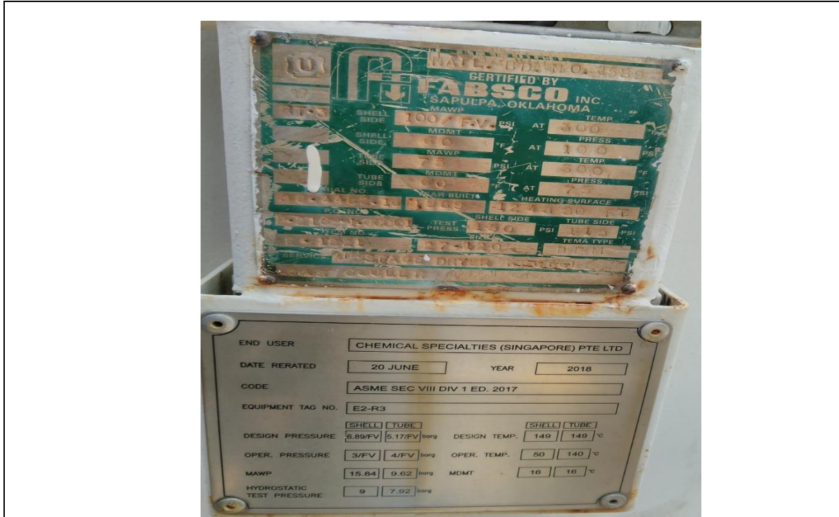
Photo 1: Name plate observed in satisfactory condition.
