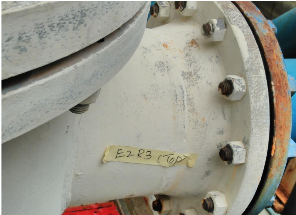
Photo 8: Top shell nozzle was in satisfactory condition
