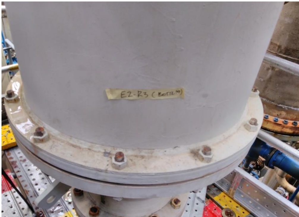
Photo 4: Bottom shell & channel flange joint were in satisfactory condition
