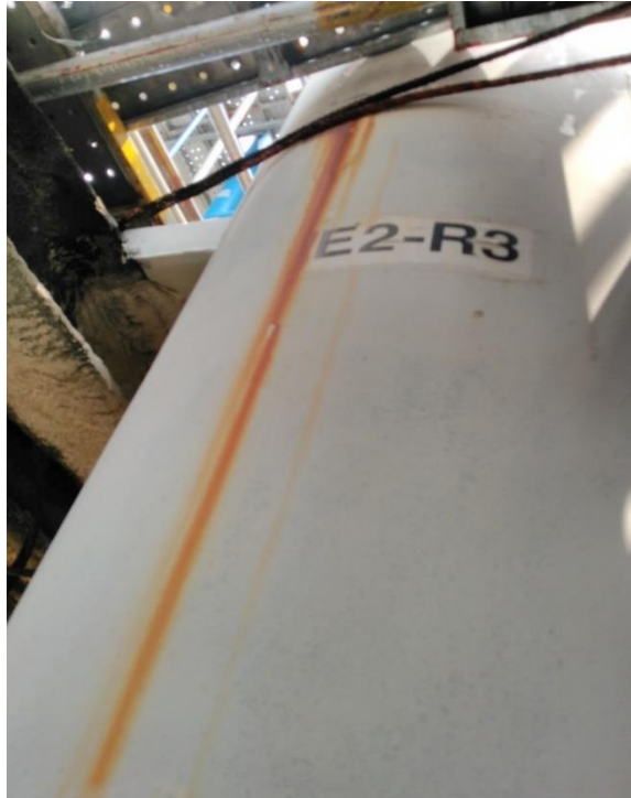
Photo 3: Shell pipe with was observed in Satisfactory condition in general. One location got minor rusting from the material in contact with the shell.
