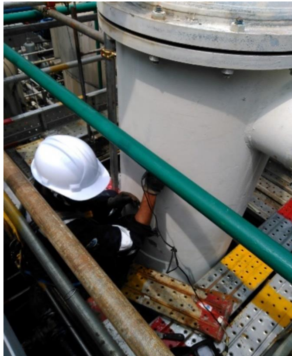
Photo 9: Top shell nozzle was observed in satisfactory condition.
