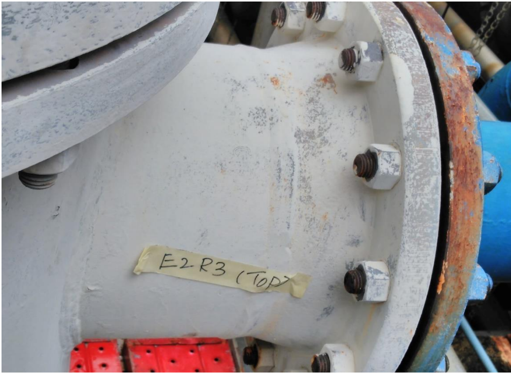
Photo 9: Top shell nozzle was observed in satisfactory condition.
