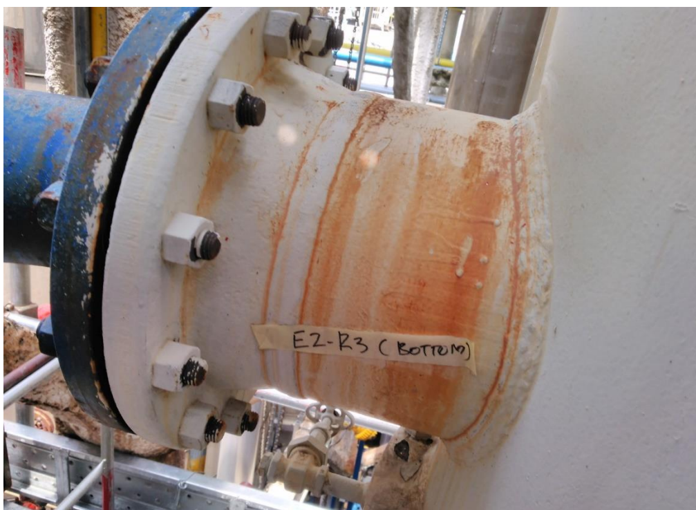
Photo 5: Bottom shell nozzle was in satisfactory condition with rust bleeding
