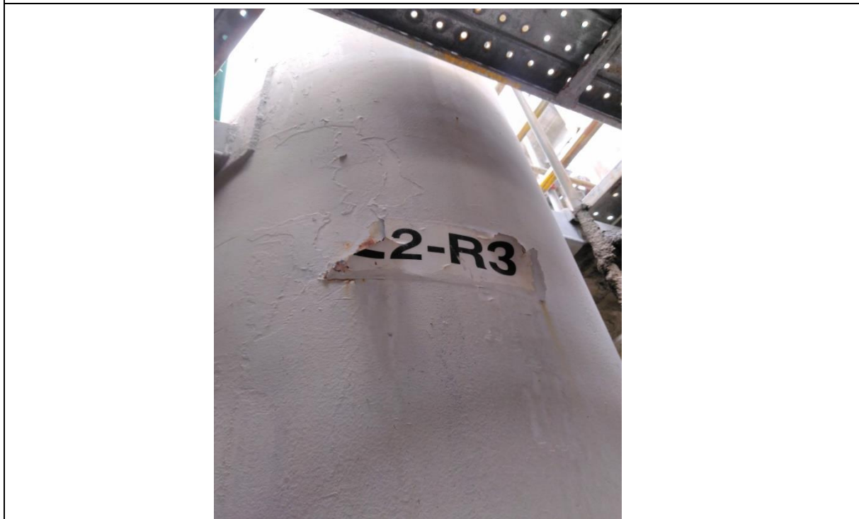
Photo 2: Shell with was observed in Satisfactory condition with coating
