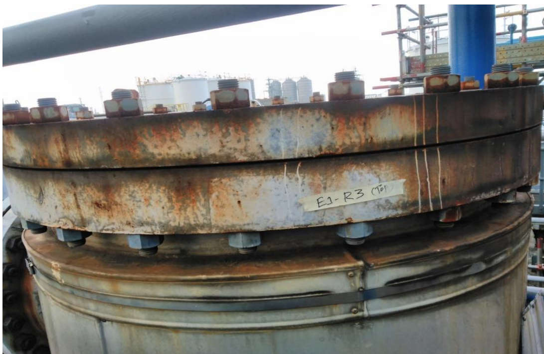
Photo 17: Top area Nozzle was observed in satisfactory condition
