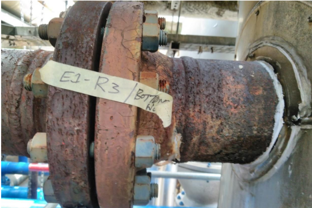
Photo 5: Bottom Shell nozzle were observed with minor corrosion
