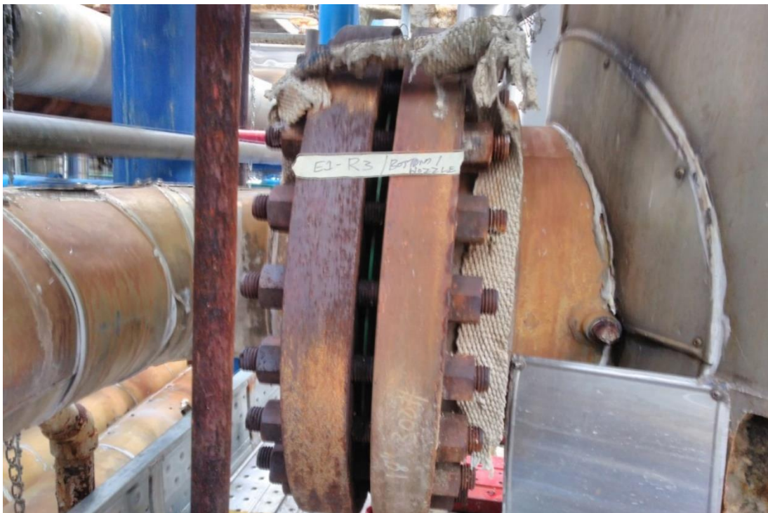
Photo 6: Bottom Shell nozzle were observed with minor rusting
