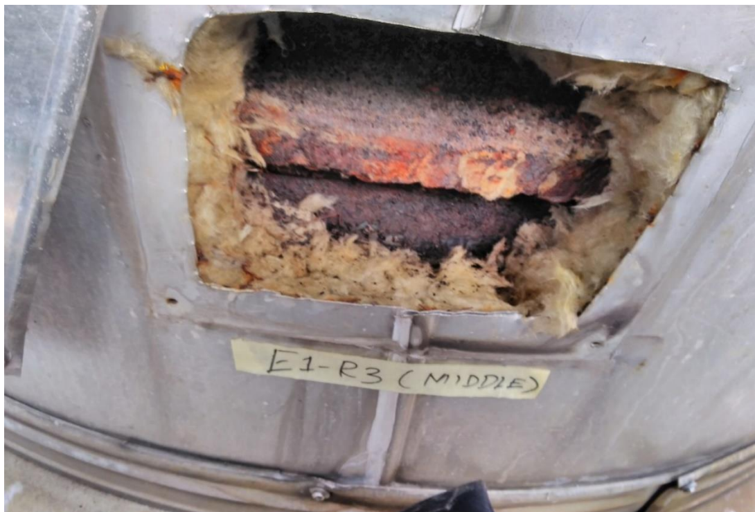
Photo 9: Middle Shell was observed with minor rust through the insulation window
