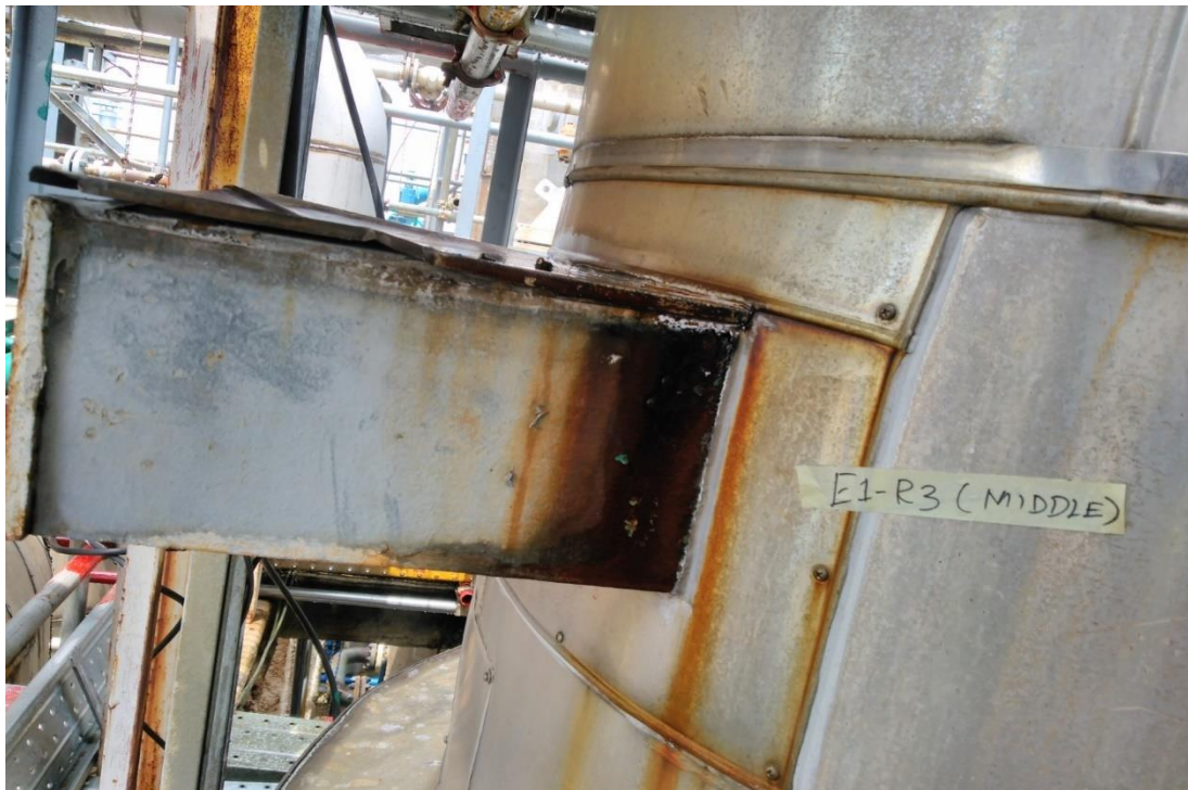
Photo 12: Support bracket was observed in satisfactory condition
