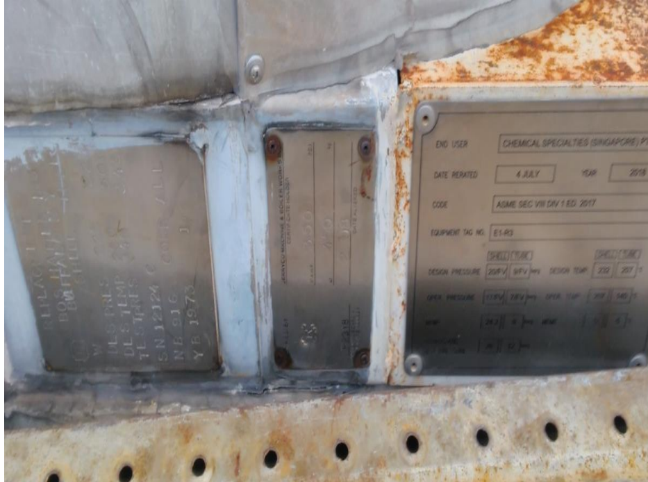
Photo 3: Tank identification plate was observed in satisfactory condition
