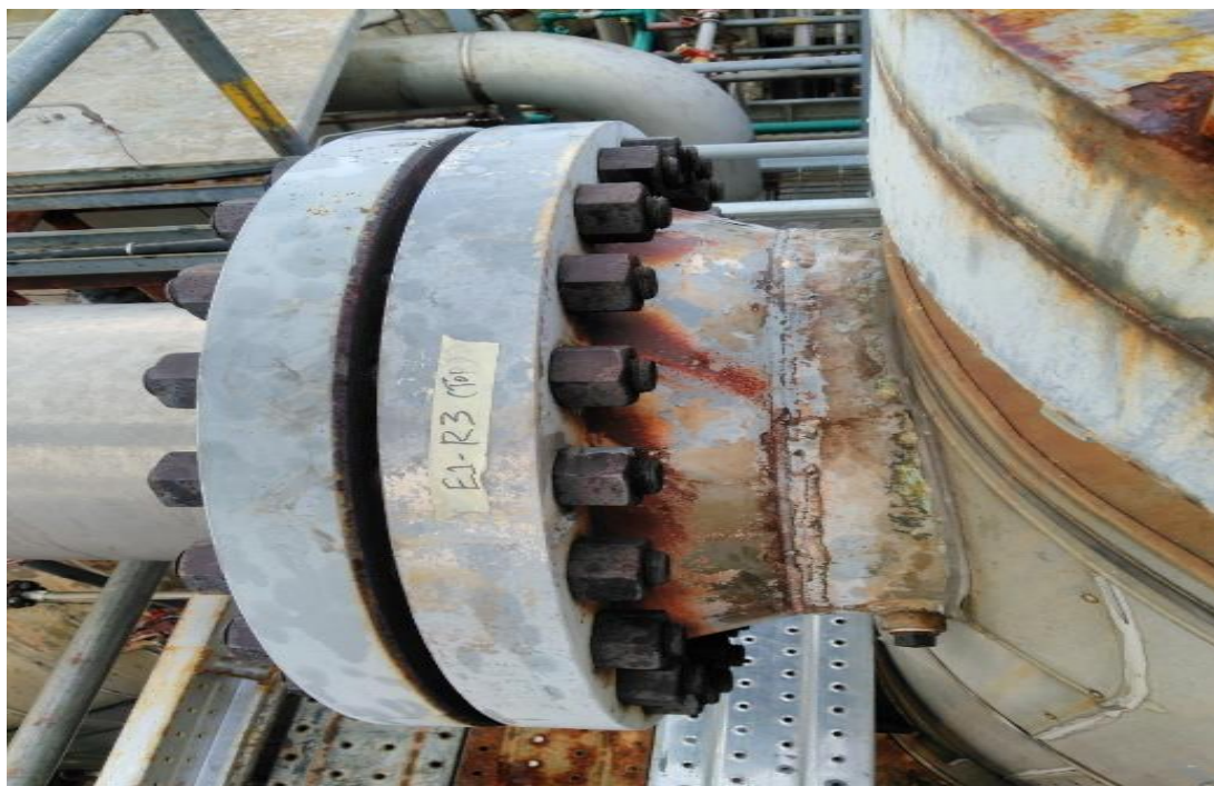
Photo 18: Top area Nozzle was observed in satisfactory condition
