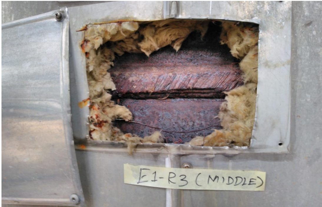
Photo 13: Middle Shell was observed with rust through the insulation window
