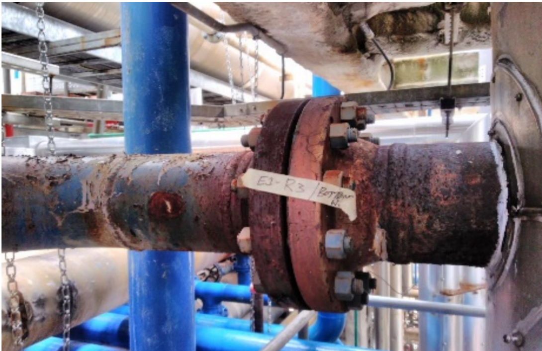
Photo 4: Bottom Shell nozzle were observed with minor corrosion
