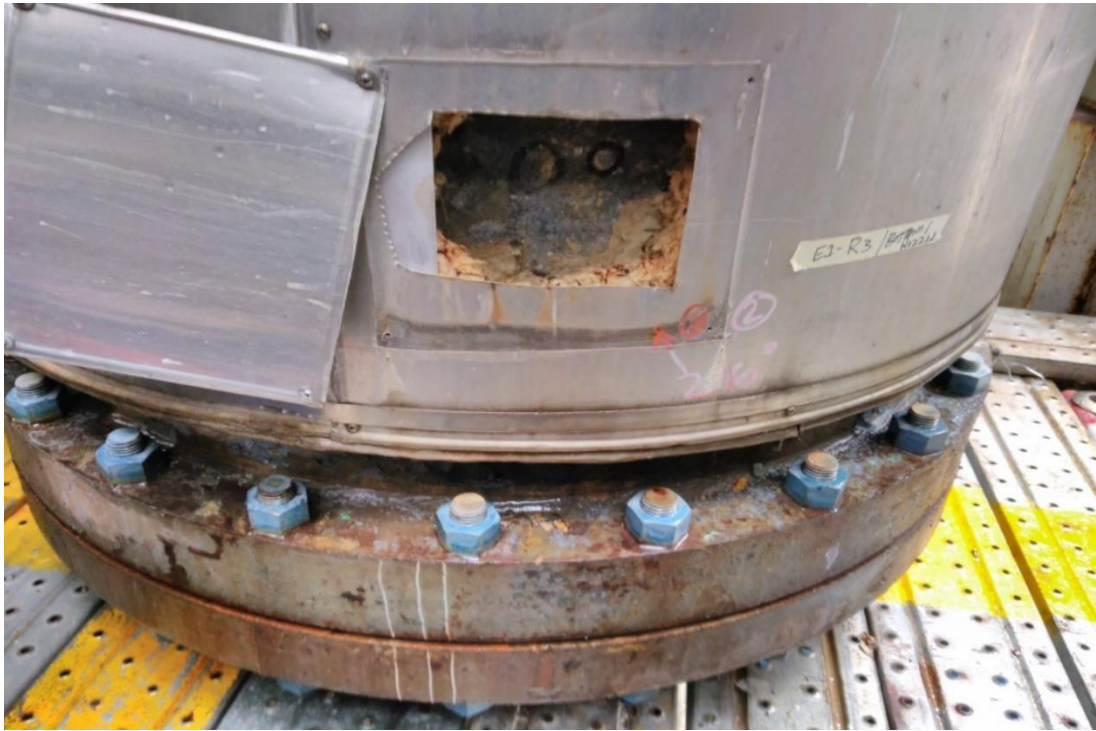
Photo 7: Bottom Shell was observed in satisfactory condition through the insulation window
