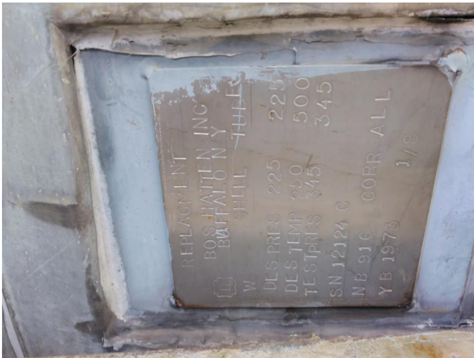
Photo 2: Design Identification plate was observed in satisfactory condition
