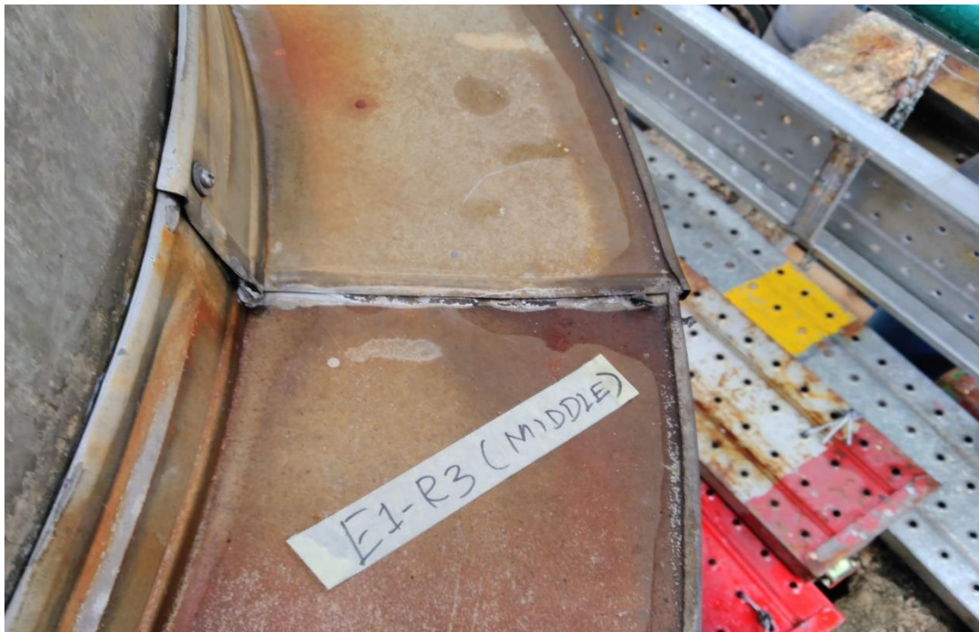
Photo 14: Flange attachment was in satisfactory condition
