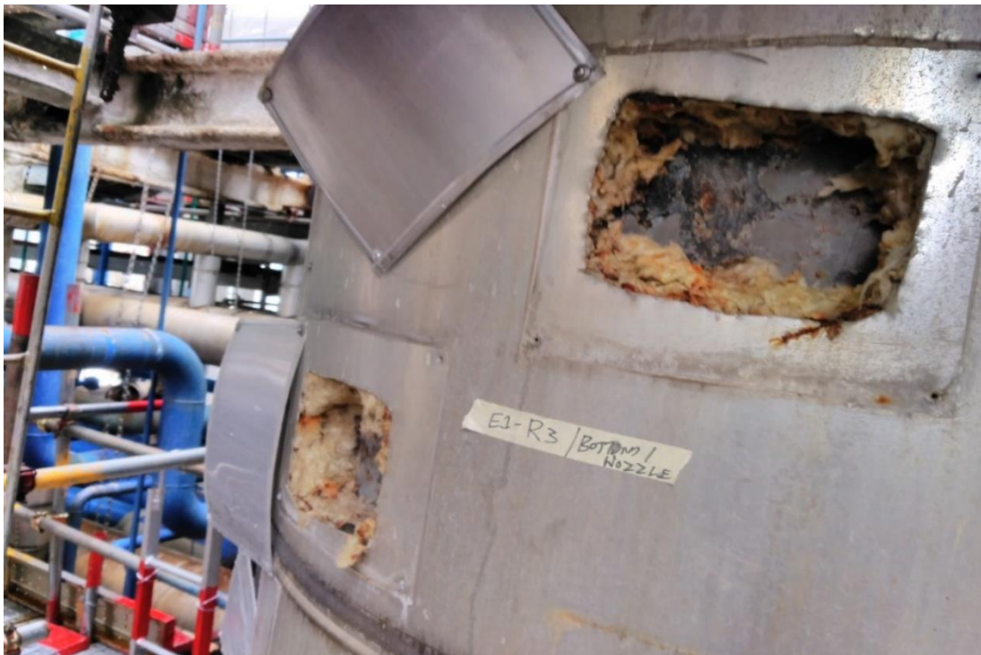
Photo 8: Bottom Shell was observed in satisfactory condition through the insulation window
