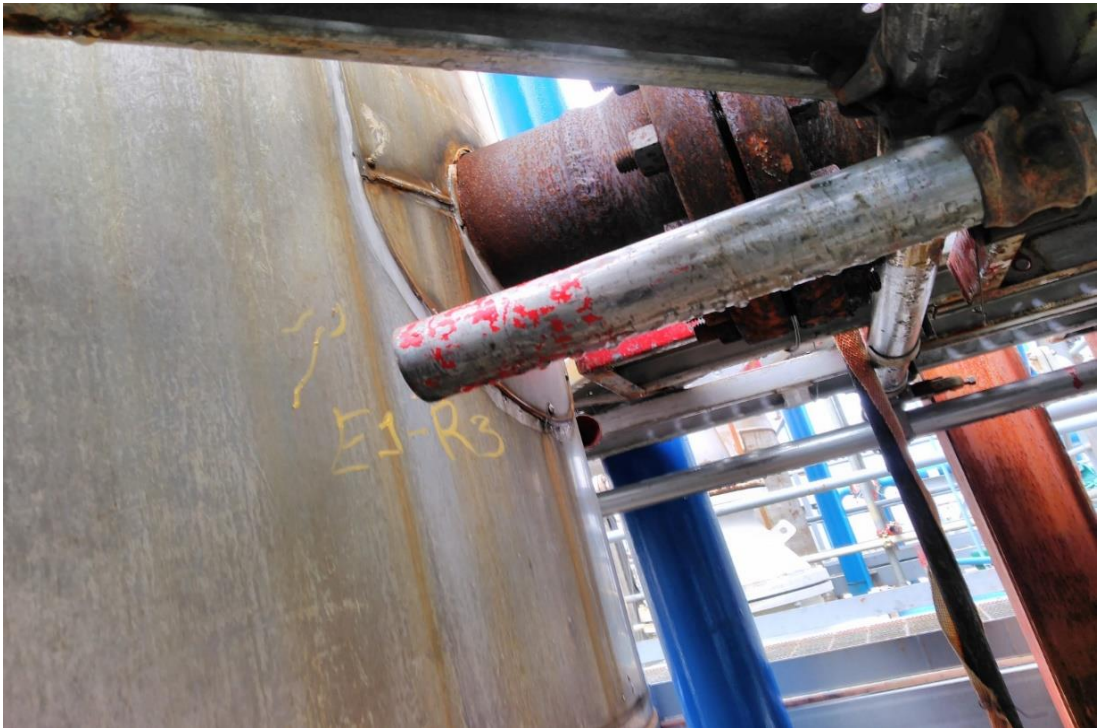
Photo 11: Shell Nozzle was observed with minor rust.
