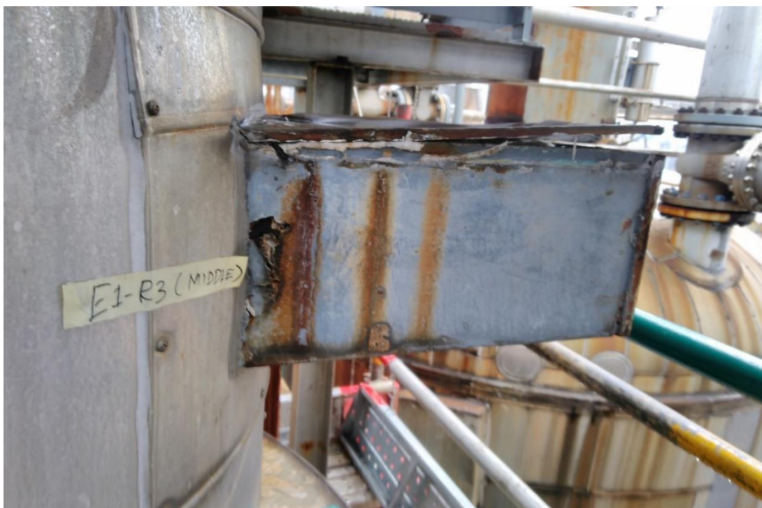
Photo 10: Support Bracket was noticed in damaged condition.
