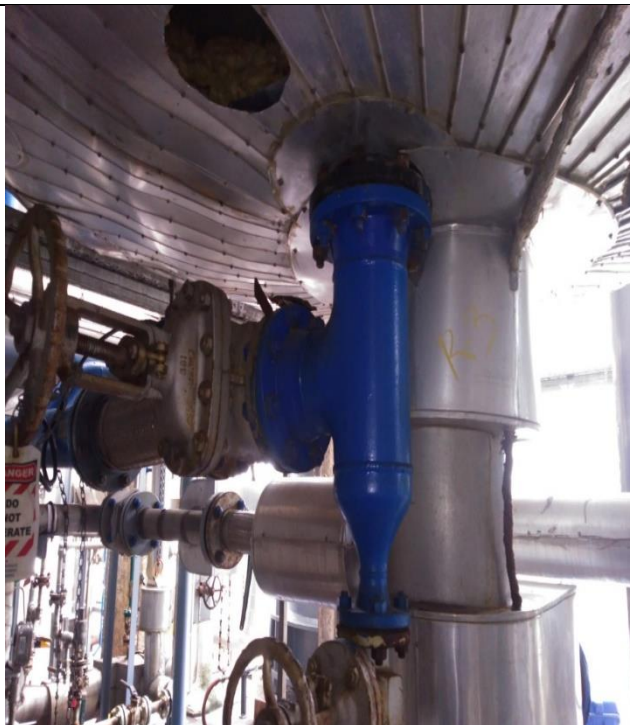
Photo 5: UTG measurement in Shell plates/ water jacket was done. External insulation was in satisfactory condition.
