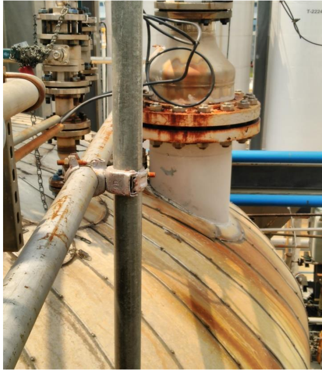
Photo 13: Top Shell nozzle was observed in satisfactory condition. Minor rust was observed on flange area.
