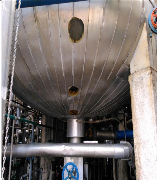
Photo 7: Bottom dish head/ water jacket was observed in satisfactory condition
