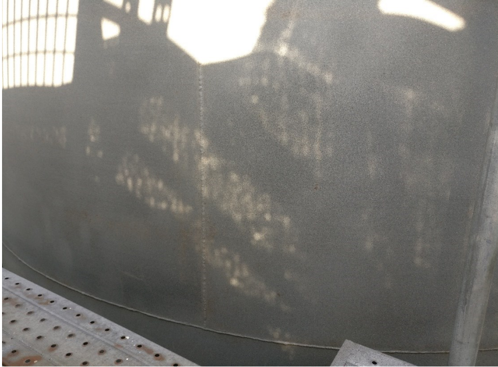
Photo 5: Tank shell external was observed with general uniform pitting. Please refer to the pitting report for details of pit depth for each shell course.
