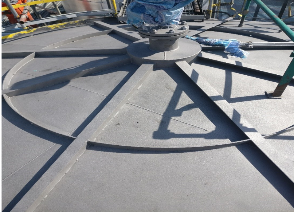
Photo 1: Roof plate and nozzle was in satisfactory condition.
