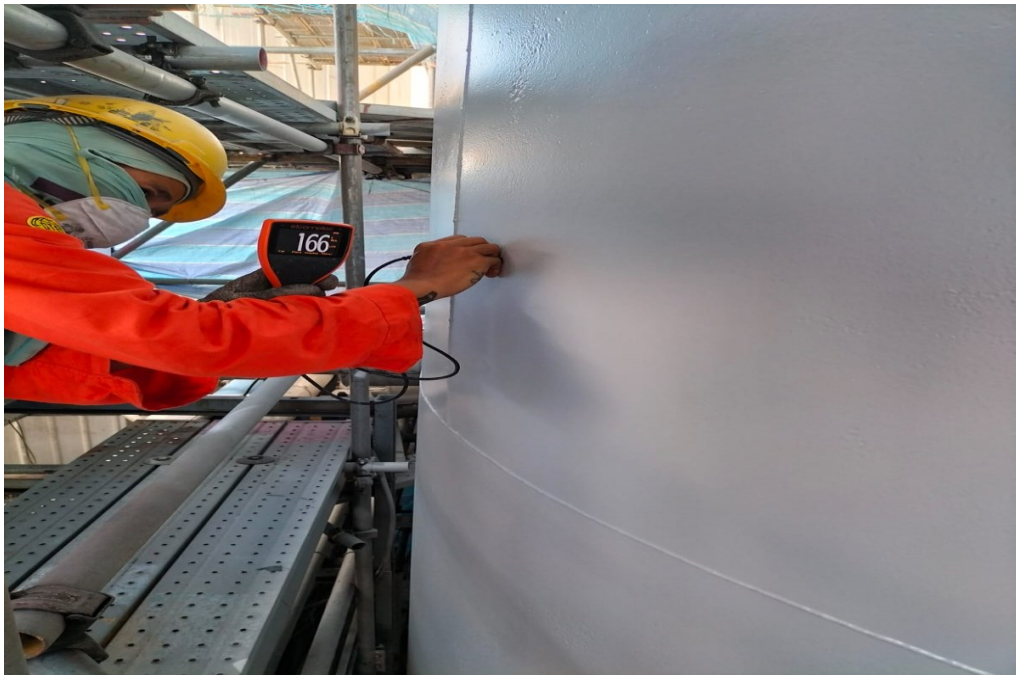
Photo 6: Tank shell external was observed with general uniform pitting. Please refer to the pitting report for details of pit depth for each shell course. External coating (new) condition was satisfactory. Photograph showing after painting and DFT measurements.
