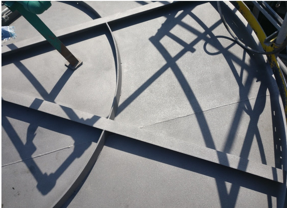
Photo 2: Roof plate was in satisfactory condition.
