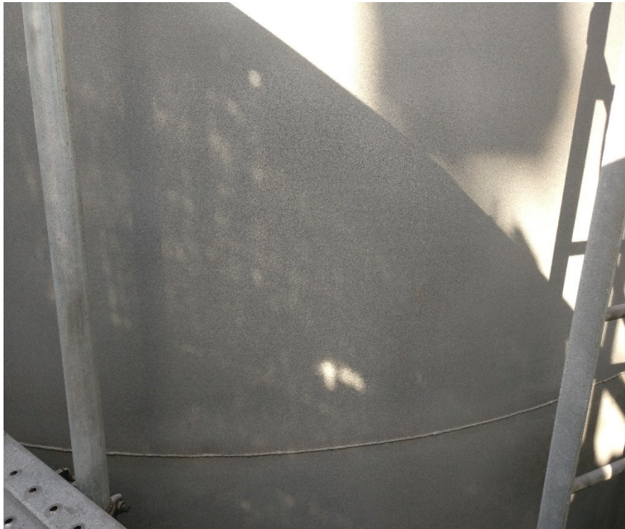
Photo 4: Tank shell external was observed with general uniform pitting. Please refer to the pitting report for details of pit depth for each shell course.
