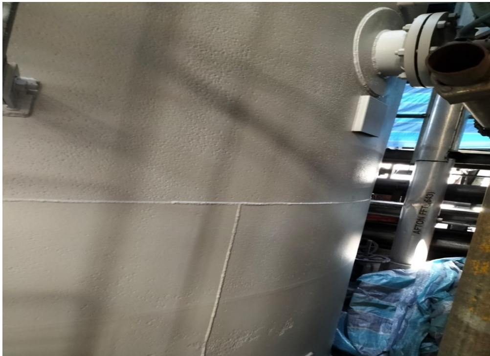
Photo 8: Tank shell external was observed with general uniform pitting. Please refer to the pitting report for details of pit depth for each shell course. External coating (new) condition was satisfactory.
