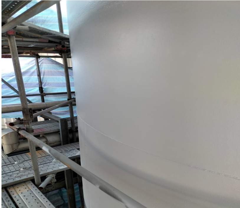
Photo 13: Tank shell external was observed with general uniform pitting. Please refer to the pitting report for details of pit depth for each shell course. External coating (new) condition was satisfactory.
